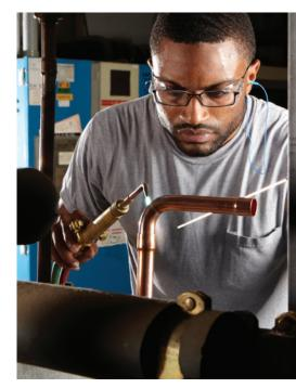
Heat broadly, and heat only the base metals – not the filler metal. Remove any toxic coatings and be careful not to overheat assemblies.
