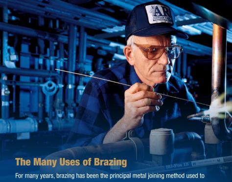
For many years, brazing has been the principal metal joining method used to fabricate heating, air conditioning and refrigeration equipment. Today, a typical HVAC unit may contain hundreds of brazed joints.
